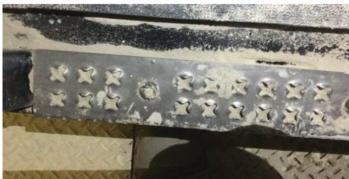
Picture 1: Dried Mud in Door Jamb
