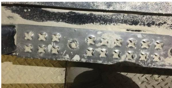
Picture 1: Dried Mud in Door Jamb
